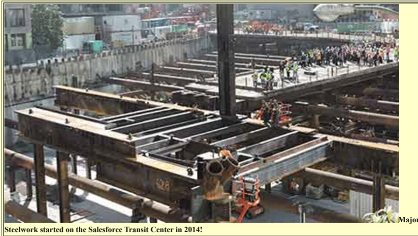
Steelwork started on the Salesforce Transit Center in 2014!
